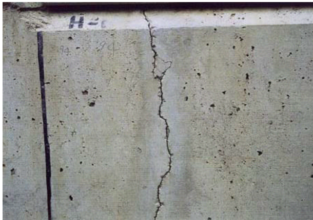
Photo.4 该该该 the crack of a concrete wall
